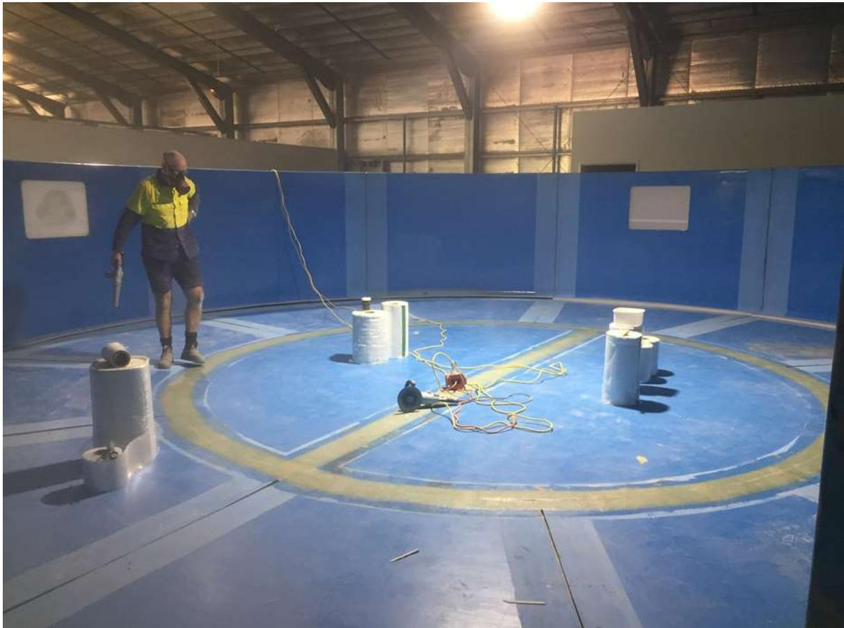
**Photo:** New 10m Diameter Tank being installed
