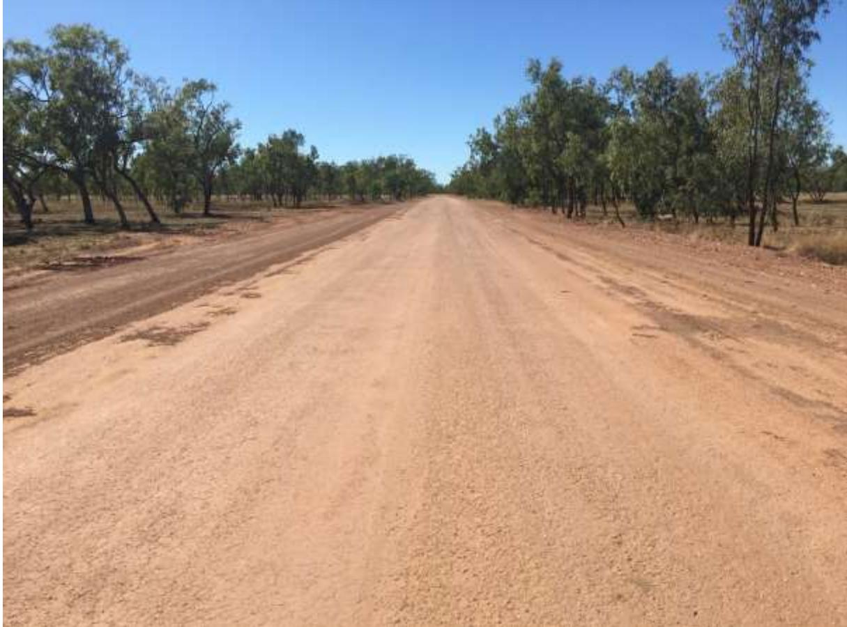
**Photo:** Completed section of subgrade works on 89B.
