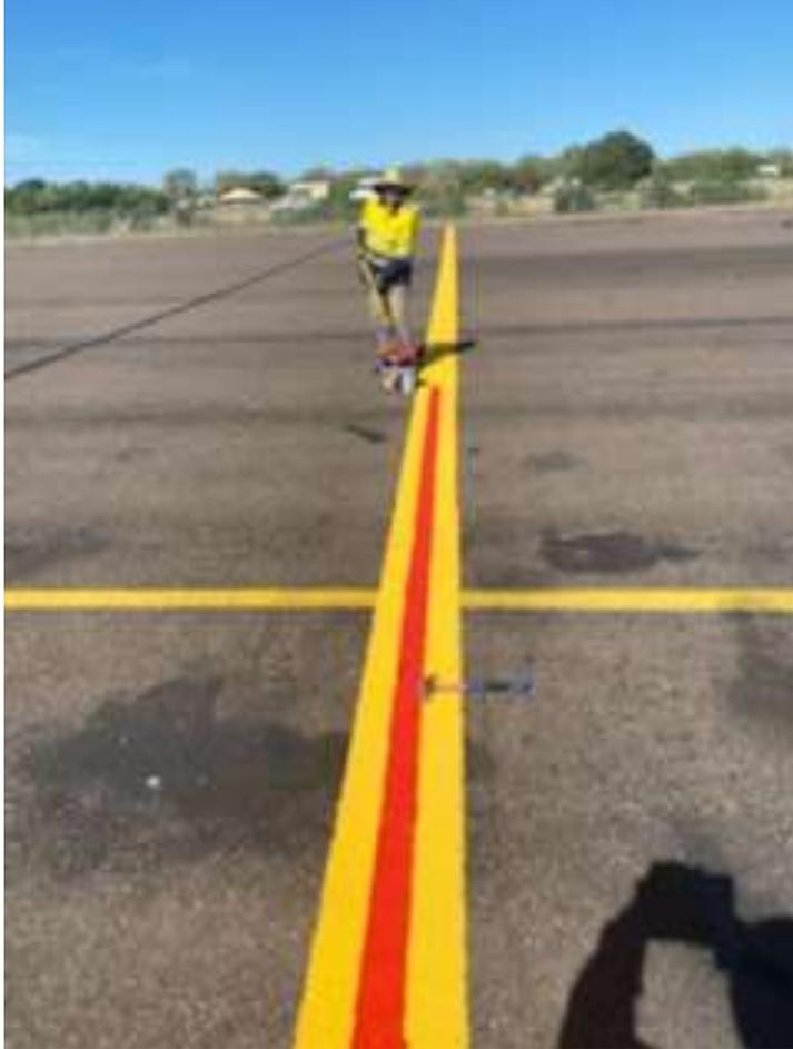
**Photo:** Linemarking the separation line between the RPT and GA apron.
