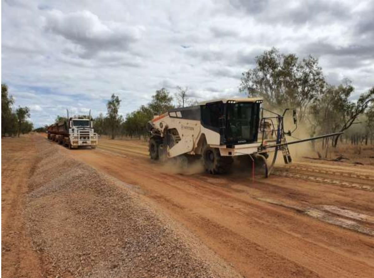
**Photo:** Stabiliser in action working on subgrade works on 89B.
