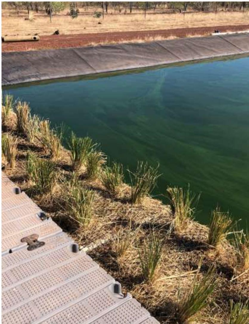
**Figure 4: Normanton STP vetiver grass pontoons**
