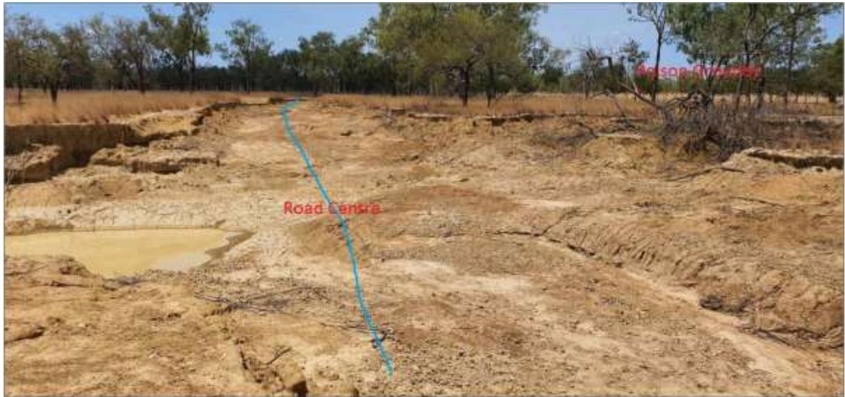
**Photo:** Erosion of road centre line
