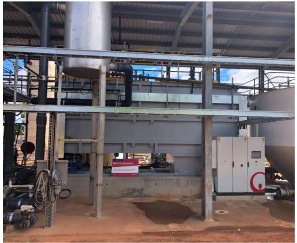
Figure 3: Actiflo Clarifier at Normanton Water Treatment Plant side view.
