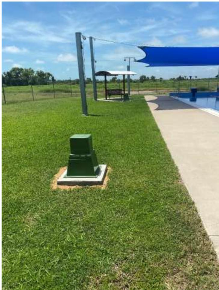
**Photo:** New turrets at the Karumba pool – before they just had some timber over the existing electrical pits
