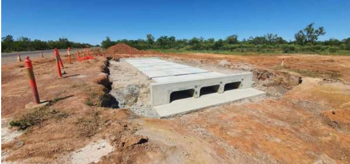
**Photo:** Installing culverts at the Lilyvale intersection
