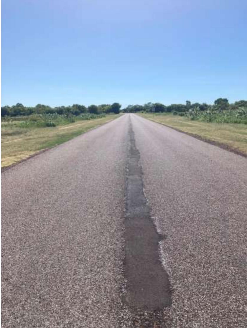
**Photo:** Pot hole patching on Col Kitching Drive
