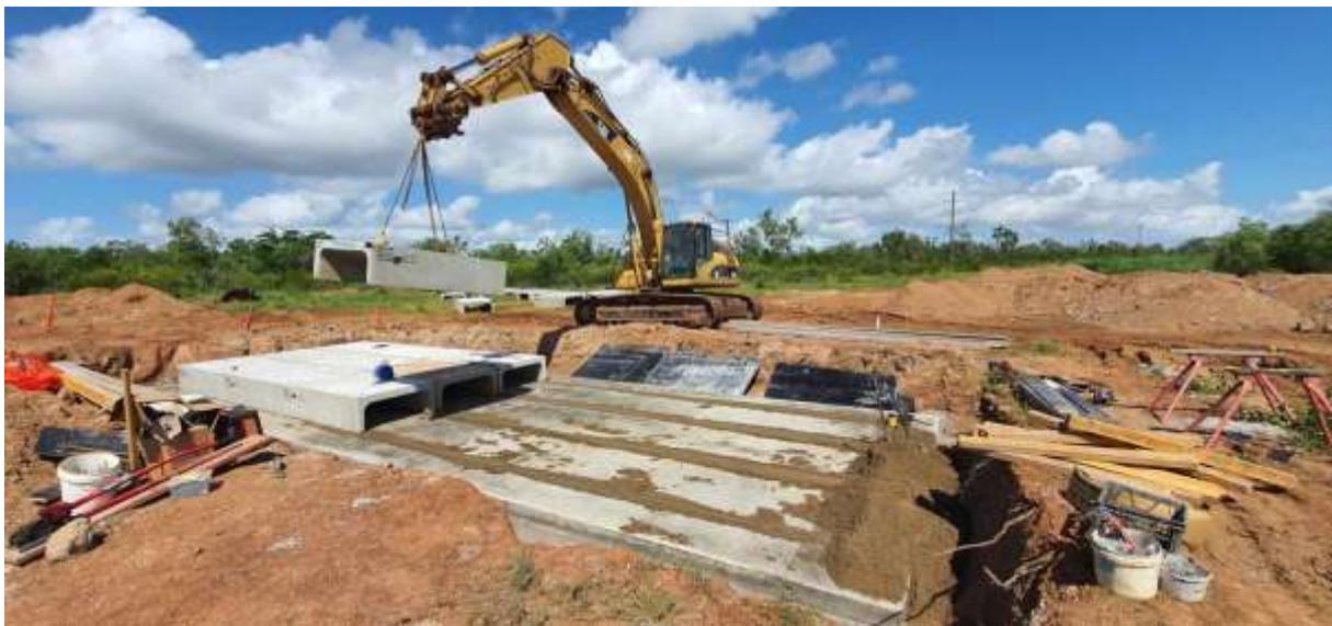
**Photo:** Installing culverts at the Lilyvale intersection
