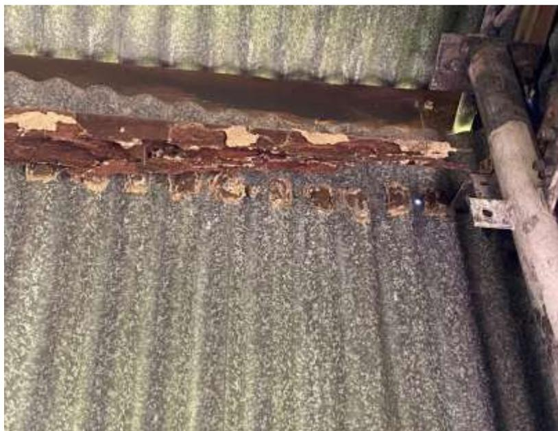
The overall flooring and main structure looks in good order, it is only the timber framework that needs replacing.
