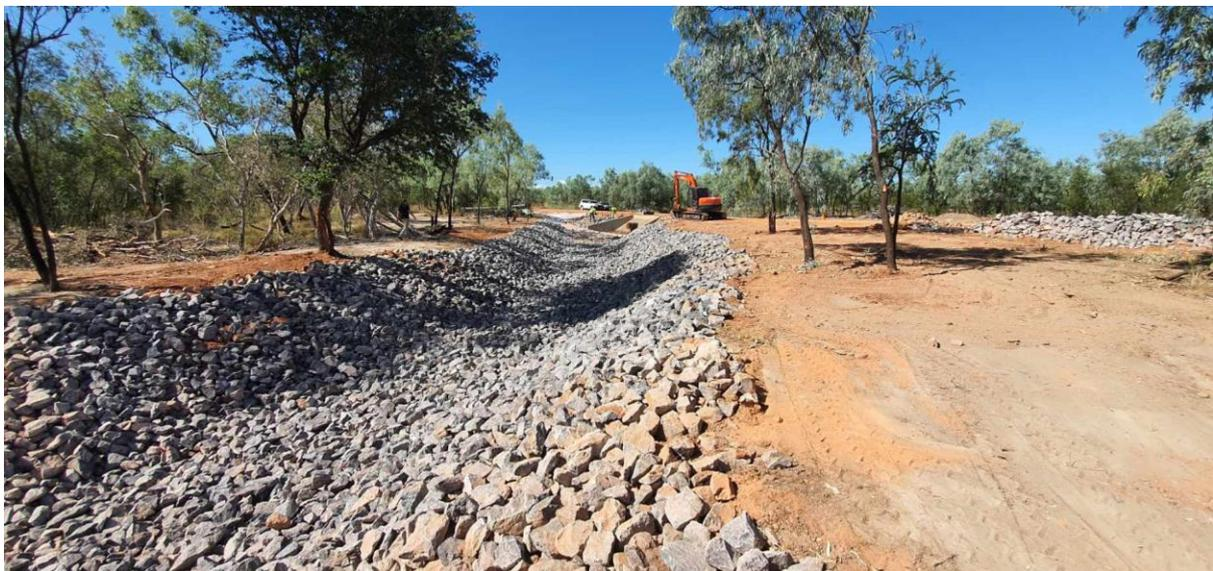
**Photo:** Rock Protection works at drain before Glenore weir
