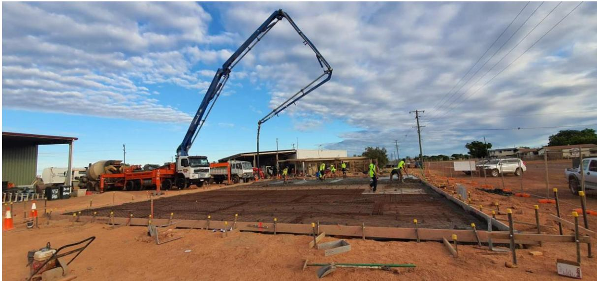
**Photo:** Pouring concrete at the Disaster Coordination Centre
