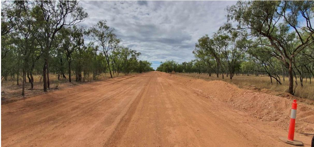
**Photo:** 89B – Emergent Works around Bayswater - spreading gravel out onto boggy sections
