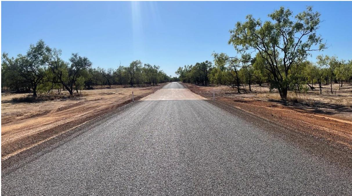
**Photo:** 89B Undertook patch repair at floodway just before Rocky Creek
