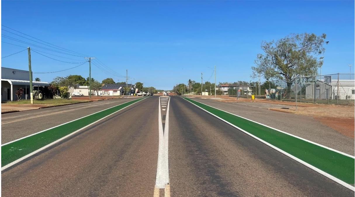
**Photo:** Completed line marking at the refuge crossing.
