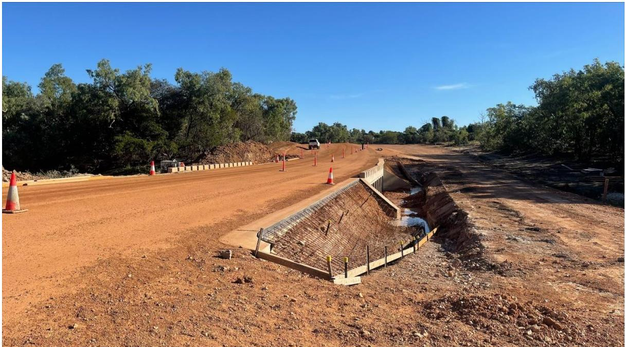
**Photo:** Armstrong Ck – completing concrete batter protection.
