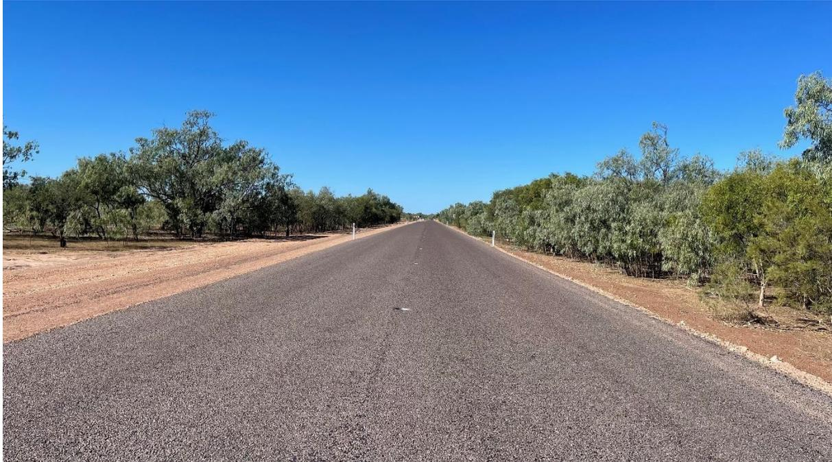
**Photo:** Completed first coat seal on the Corduroy Crossing.
