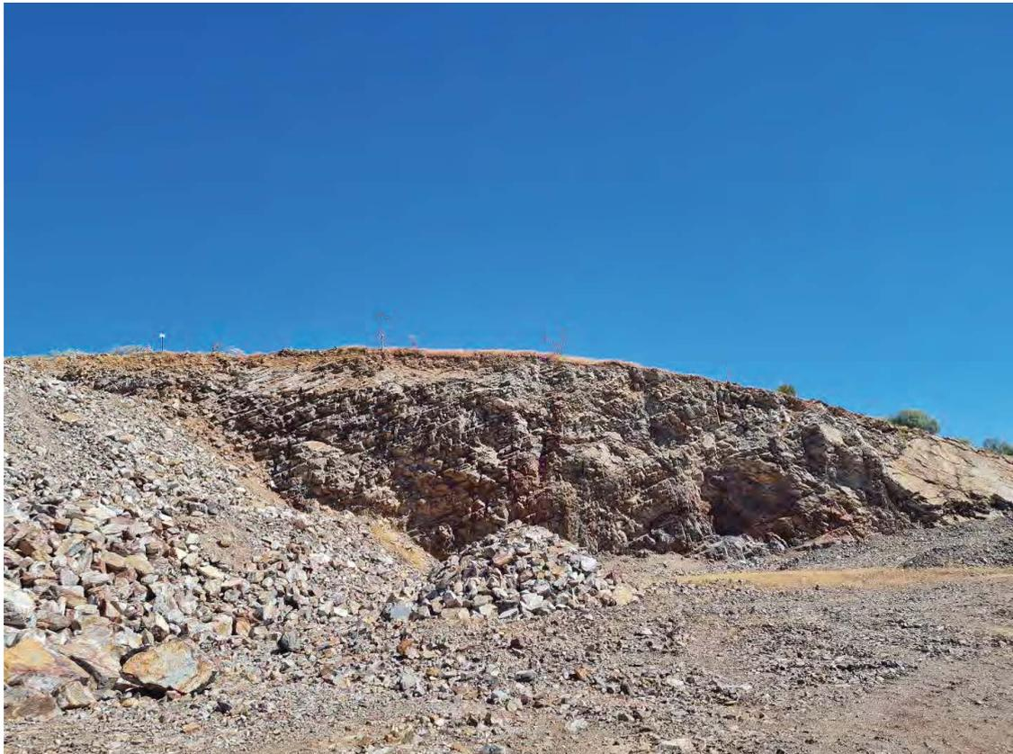
Figure 6-8: Jubilee Quarry current working face - heavily fractured and not suitable for rock armour.
