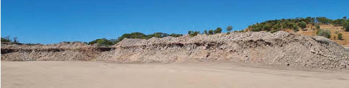
Figure 6-5: Jubilee Quarry overburden stockpile, currently sorted for rock supply.
