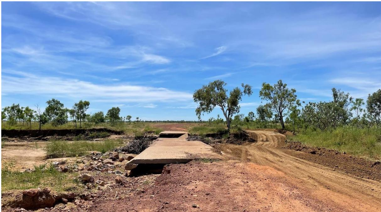
**Photo** – Damage on the Bore Drain Creek Causeway on the Burketown Road
