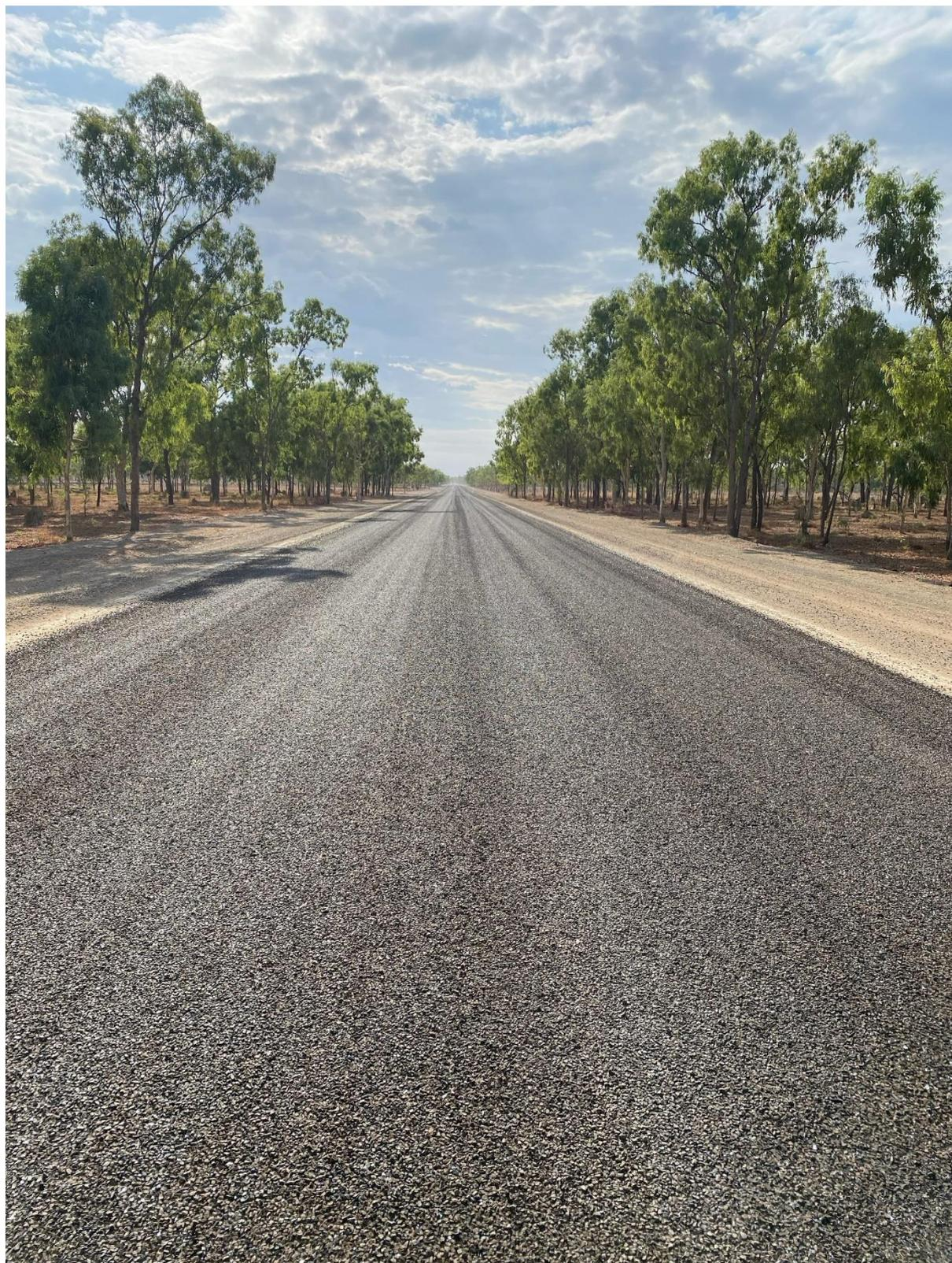
**Photo:** Kowanyama Road Betterment Works - 5km completed two coat bitumen seal project
