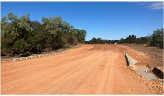
Culverts installed. Right hand side of image shows old road
