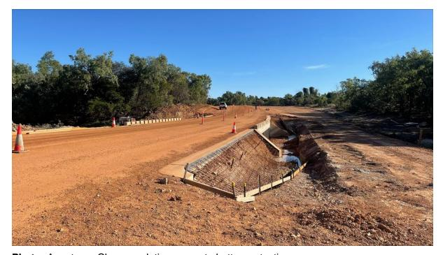
**Photo:** Armstrong Ck – completing concrete batter protection.
