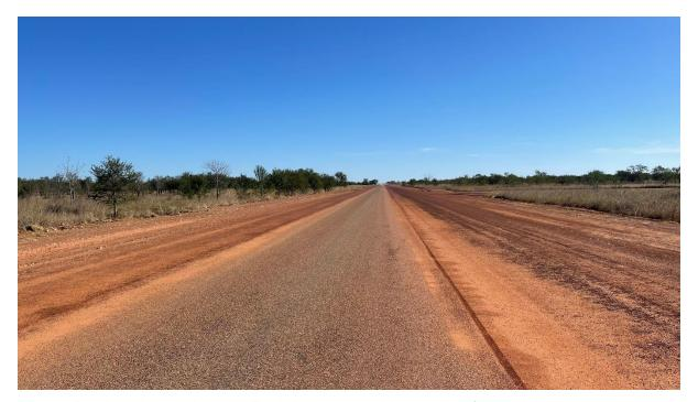
Photo: Patchwork completed at Fools Lagoon awaiting sealing for 24 July
