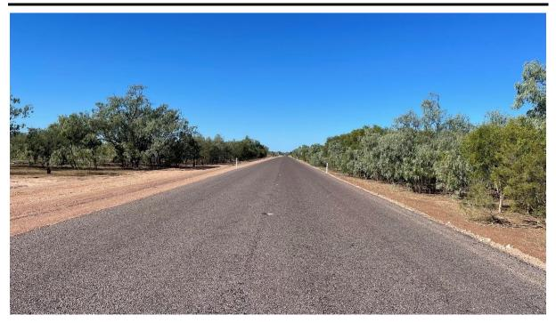
**Photo:** Completed first coat seal on the Corduroy Crossing.
