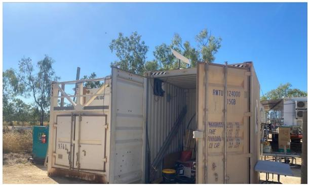
Figure 3 - Camp Container with Starlink attached to the roof and power supply inside
