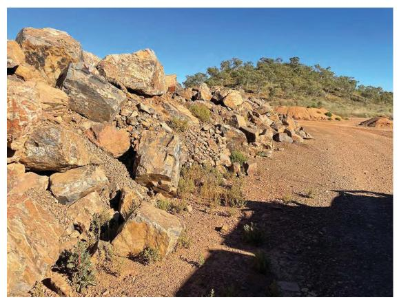
Figure 6-18: Stockpile of oversized rock armour.
