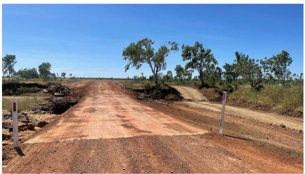
Photo – Emergent Works on the Bore Drain Creek Causeway on the Burketown Road
