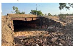
The stone culverts, kerb and channel date from the 1880s, early in the town's settlement. They were constructed from stone from the Normanton Quarry located behind the hospital. The gutters start at the Burns Philp Building and can be seen either side of Landsborough Street to the Westpac Bank.
