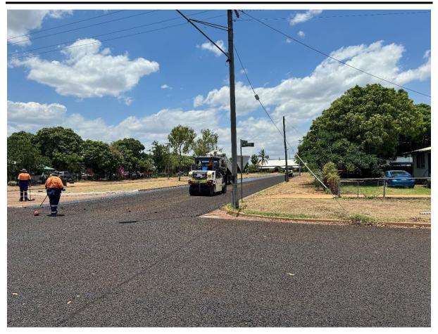
Photo: Intersection of Dutton and Balonne Street reseal
