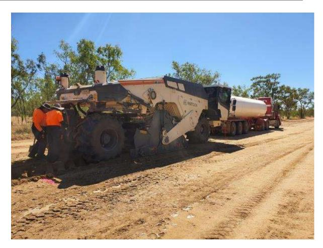
Photo: Stabiliser in action – preparing subgrade works 89B.
