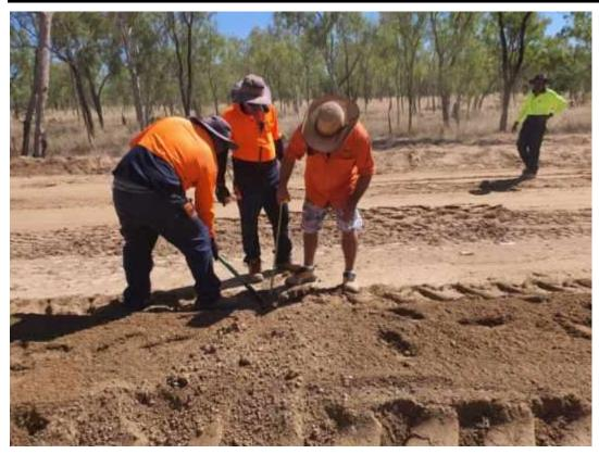
**Photo:** Checking depth of subgrade.
