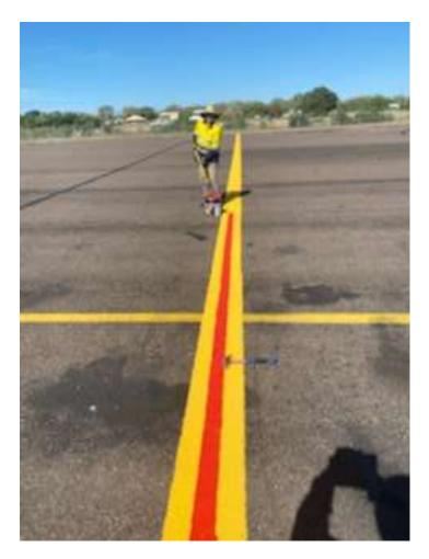
**Photo:** Linemarking the separation line between the RPT and GA apron.
