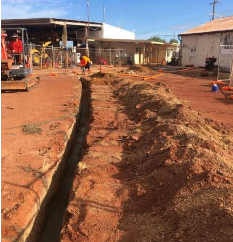
Photo: Installing electrical conduits for the Trades Shed.
