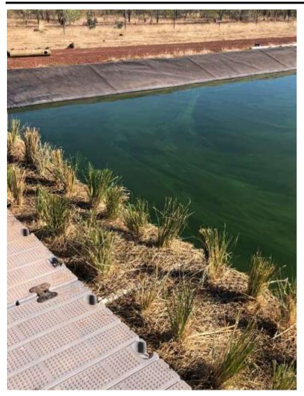
Figure 4: Normanton STP vetiver grass pontoons
