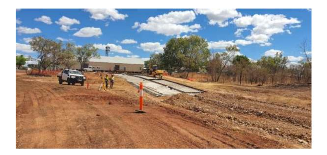
**Photo:** Preparing the ramp for concrete pour.
