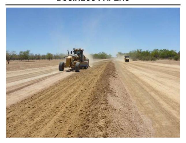
Photo: Spreading out the gravel on the Kowanyama Road.
