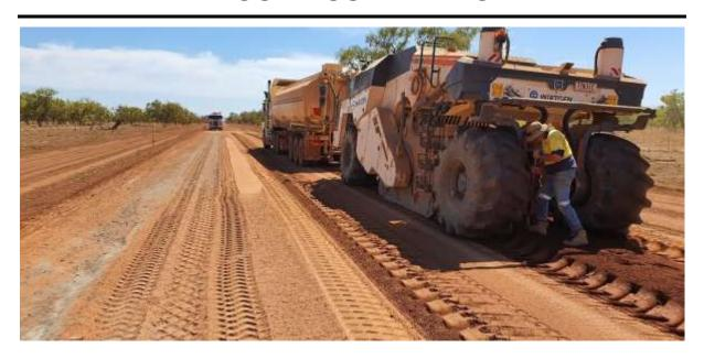
Photo: Stabilisation works on the 6km TIDS new sealing project on the Burketown Rd.
