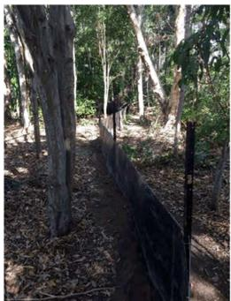
Images 20 and 21 Trench construction to bury the bottom of the fence (*left*) and the completed fence as it runs through scrub around the dam (*right*)
