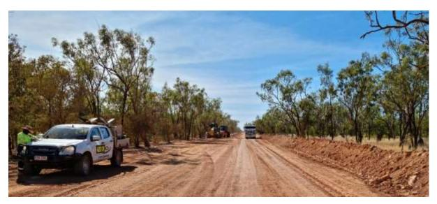
**Photo:** Laying out gravel on 5km section on 89B.
