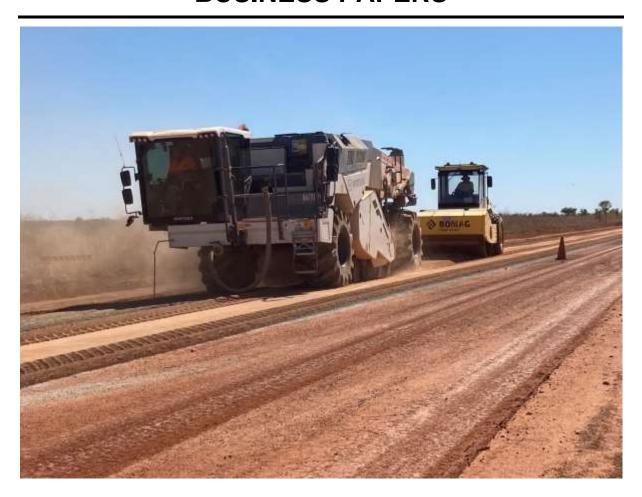
Photo: 89A Stabilisation works by Council southern end of the Flinders River section.
