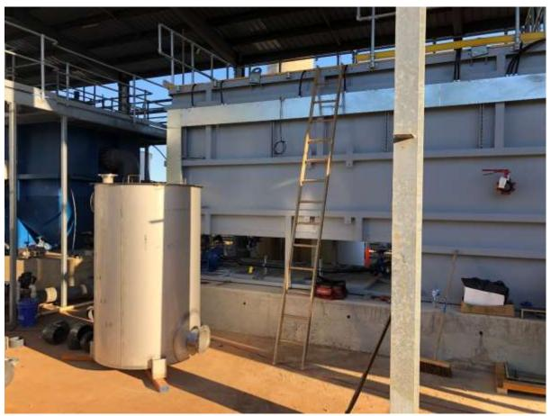
Figure 3: Actiflo Clarifier on concrete plinth at Normanton Water Treatment Plant.
