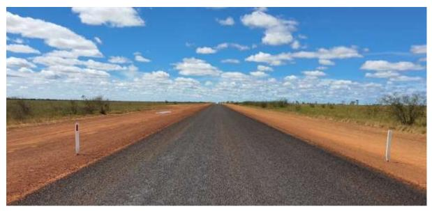
Photo: TIDS - Burketown Road - Completed sealed works at Inverleigh
