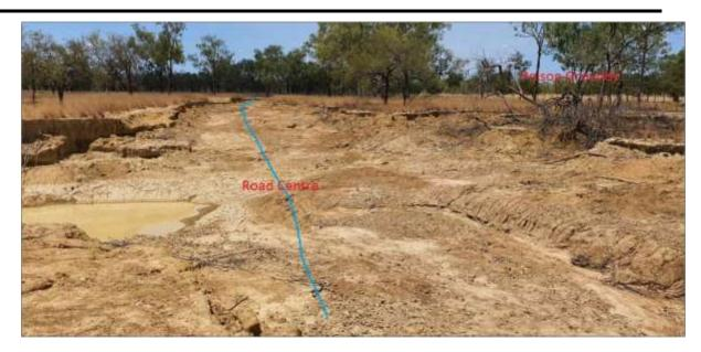
Photo: Erosion of road centre line
