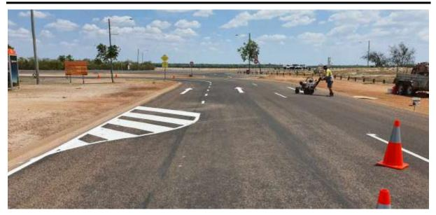
Photo: Setting out Linemarking at the Point
