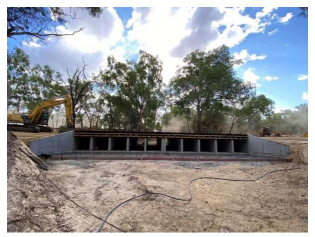
Photo: ATSITIDS - Magnificent Creek Overflow (Topsy Ck) causeway under construction
