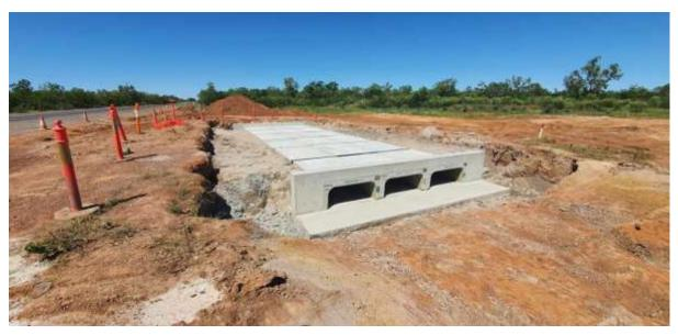
Photo: Installing culverts at the Lilyvale intersection
