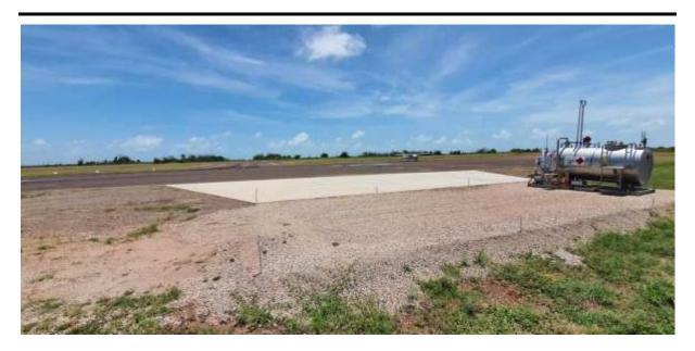
Photo: Turnaround slab constructed at Karumba Bowser
