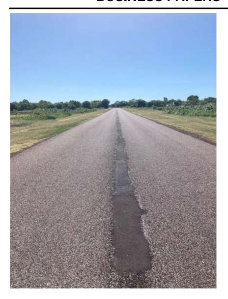
Photo: Pot hole patching on Col Kitching Drive
