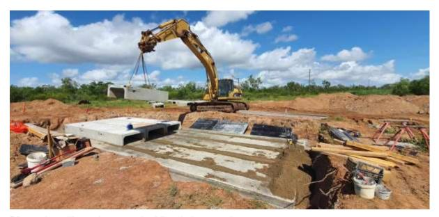
Photo: Installing culverts at the Lilyvale intersection
