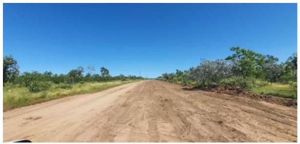
Photo: Internal Road pegged and being formed up at the Lilyvale subdivision
