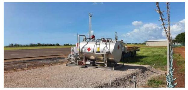
**Photo:** AVGAS Bowser installed at the Karumba Aerodrome.
