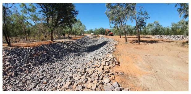
Photo: Rock Protection works at drain before Glenore weir
