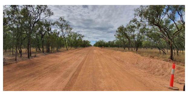
**Photo:** 89B - Emergent Works around Bayswater - spreading gravel out onto boggy sections
