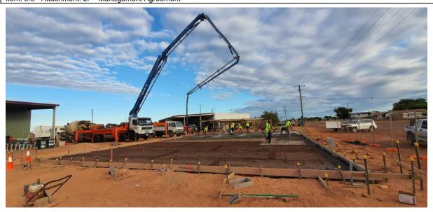
Photo: Pouring concrete at the Disaster Coordination Centre
