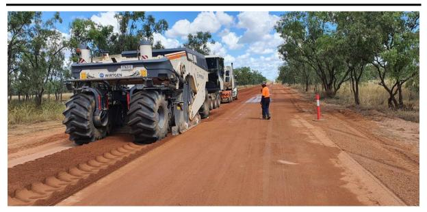
Photo: CN17937 89B Subgrade Works
