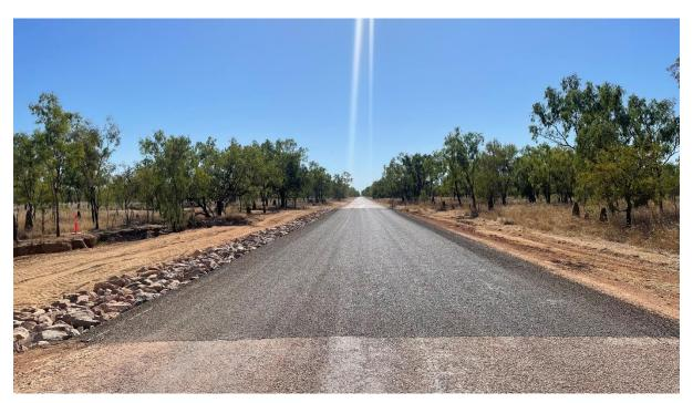
**Photo:** 89B – Completed concrete rats wall and stone pitching and patch repair work at the old seal just around the bend from the Glencoe turn-off.
