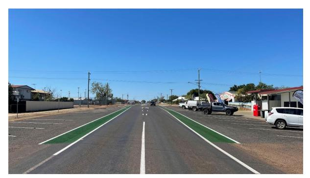
Photo: Completed line marking at the refuge crossing.
