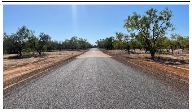
**Photo:** 89B Undertook patch repair at floodway just before Rocky Creek
