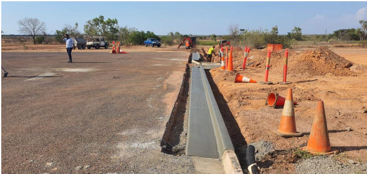
Photo: McNamara Street Kerb and Channel
