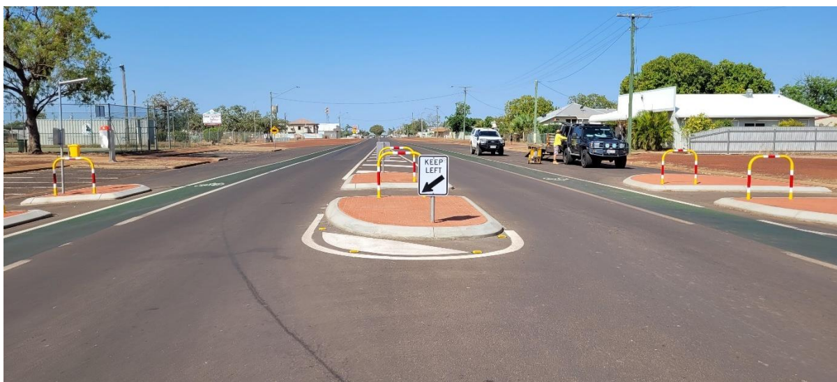
Photo: Additional cats eye installed at the pedestrian refuge
