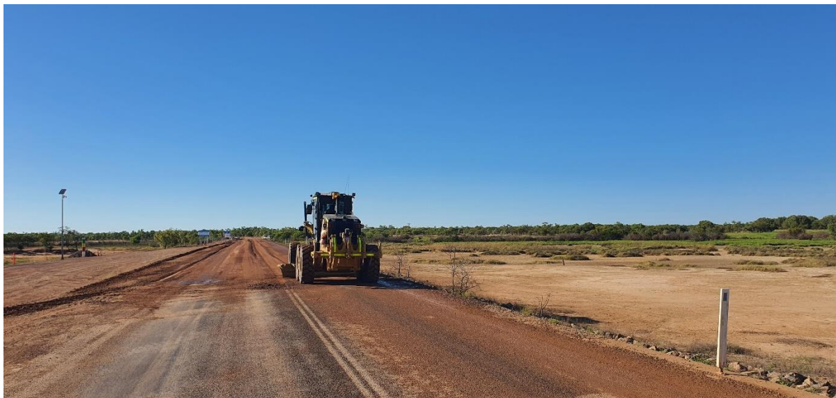
Photo: Performing final trim works on the Corduroy Crossing.
