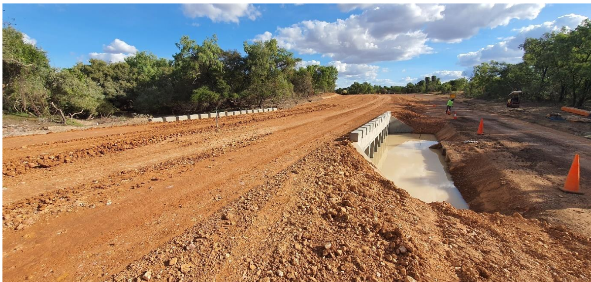
Photo: Armstrong Creek – Main Culverts installed – Old road on right
