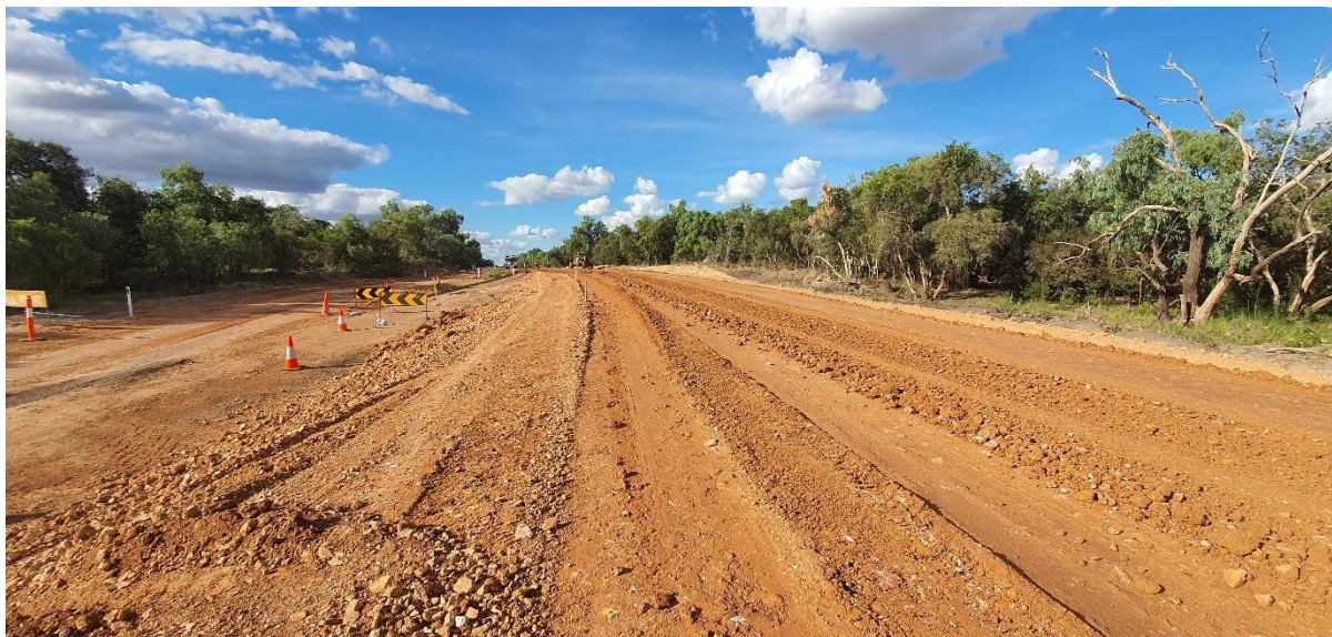
Photo: Building up the road at Armstrong Creek. Old road on the left.
