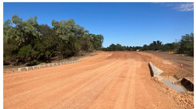
Culverts installed. Right hand side of image shows old road
