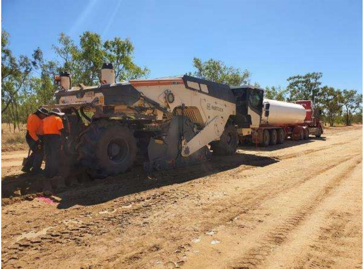
**Photo:** Stabiliser in action – preparing subgrade works 89B.
