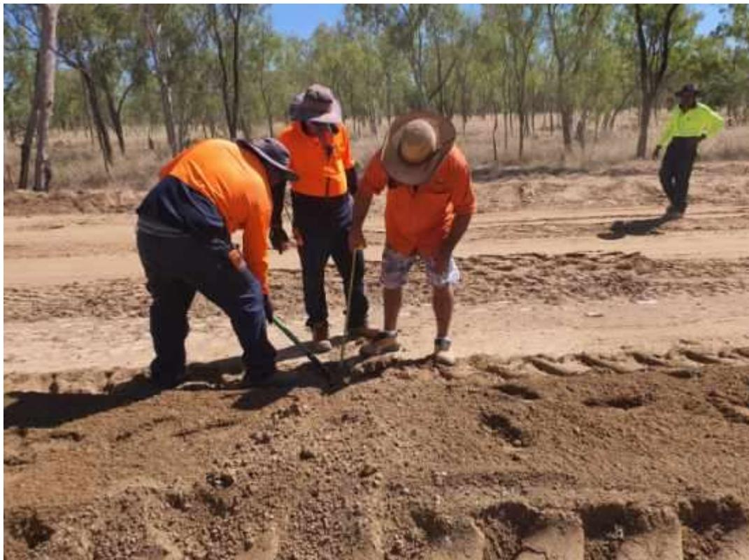
**Photo:** Checking depth of subgrade.
