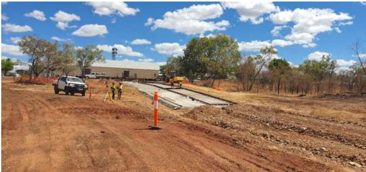
**Photo:** Preparing the ramp for concrete pour.
