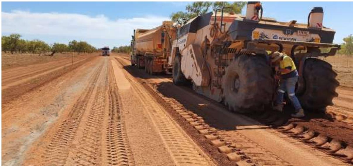
**Photo:** Stabilisation works on the 6km TIDS new sealing project on the Burketown Rd.
