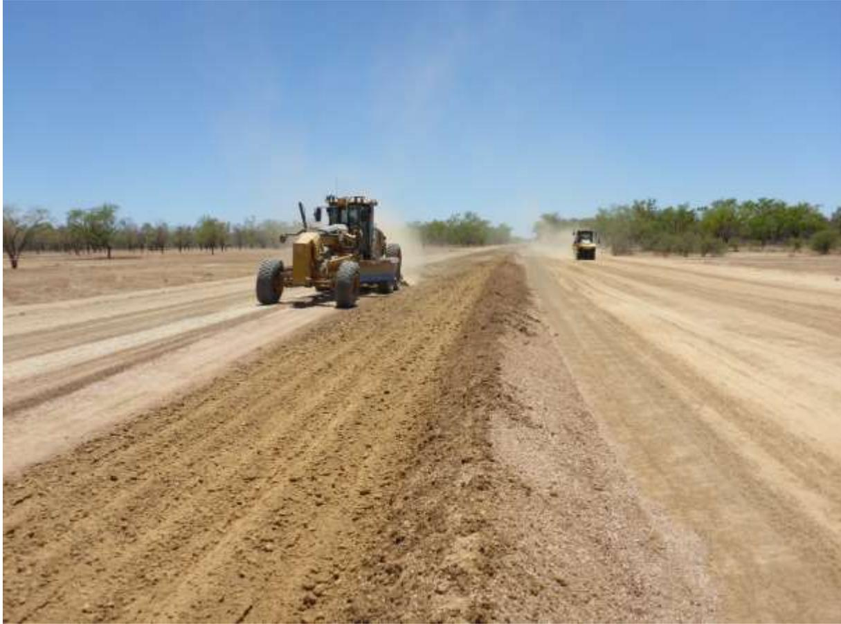
**Photo:** Spreading out the gravel on the Kowanyama Road.
