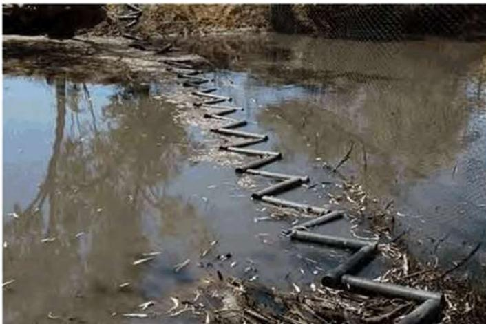
**Image 3** The new poly battens are proving to be effective for use in floodways
