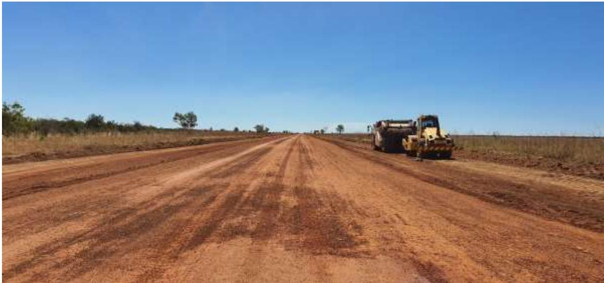
**Photo:** 89A Widening works started southern end of the Flinders River section.
