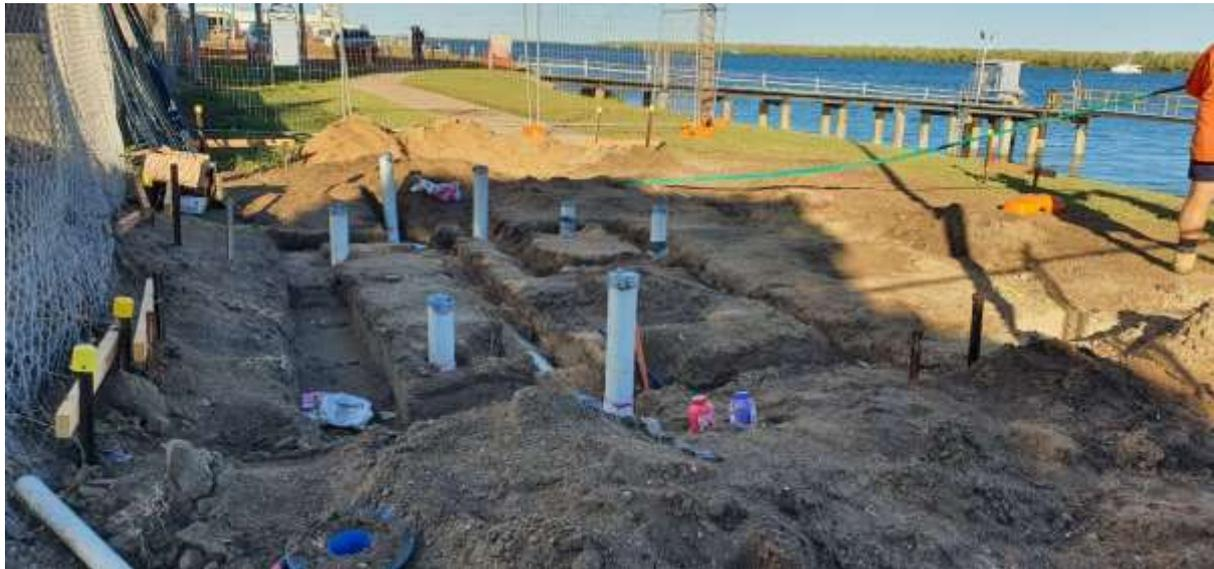
**Photo:** New toilets at the Karumba Boat Ramp – Plumbing being installed
