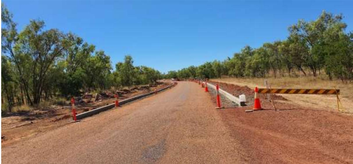
**Photo:** 89A concrete protection works southern end of the Flinders River section.
