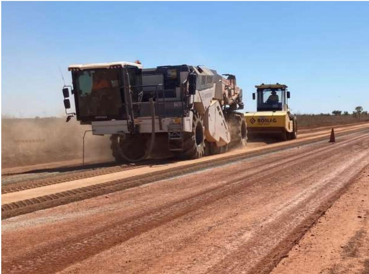
**Photo:** 89A Stabilisation works by Council southern end of the Flinders River section.
