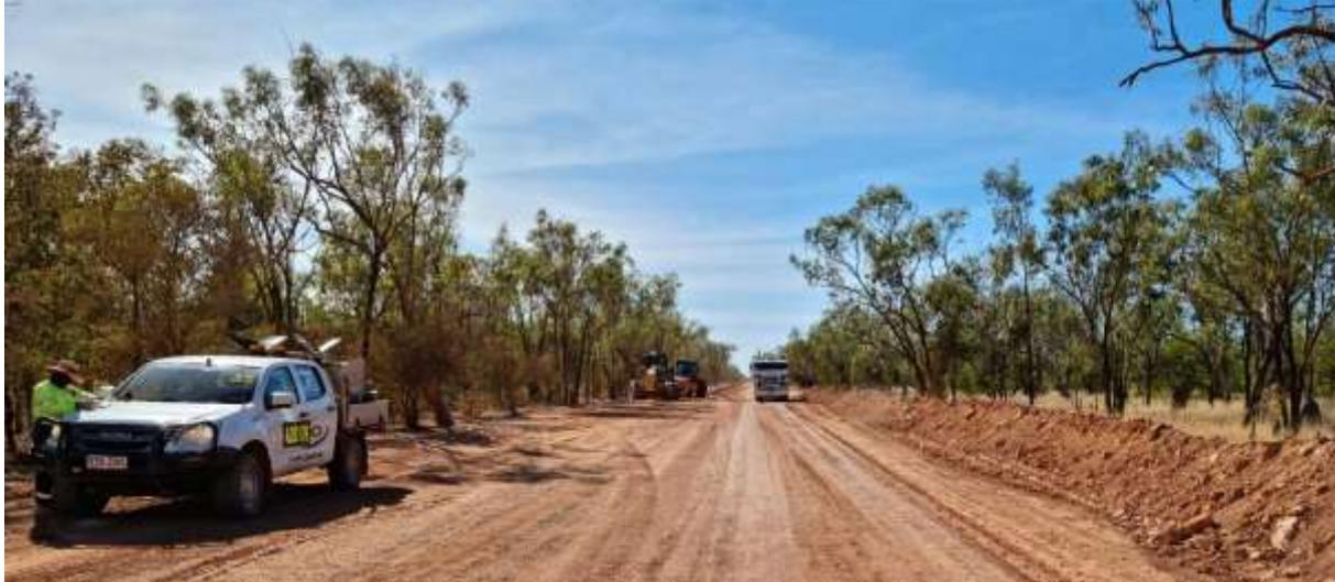
**Photo:** Laying out gravel on 5km section on 89B.
