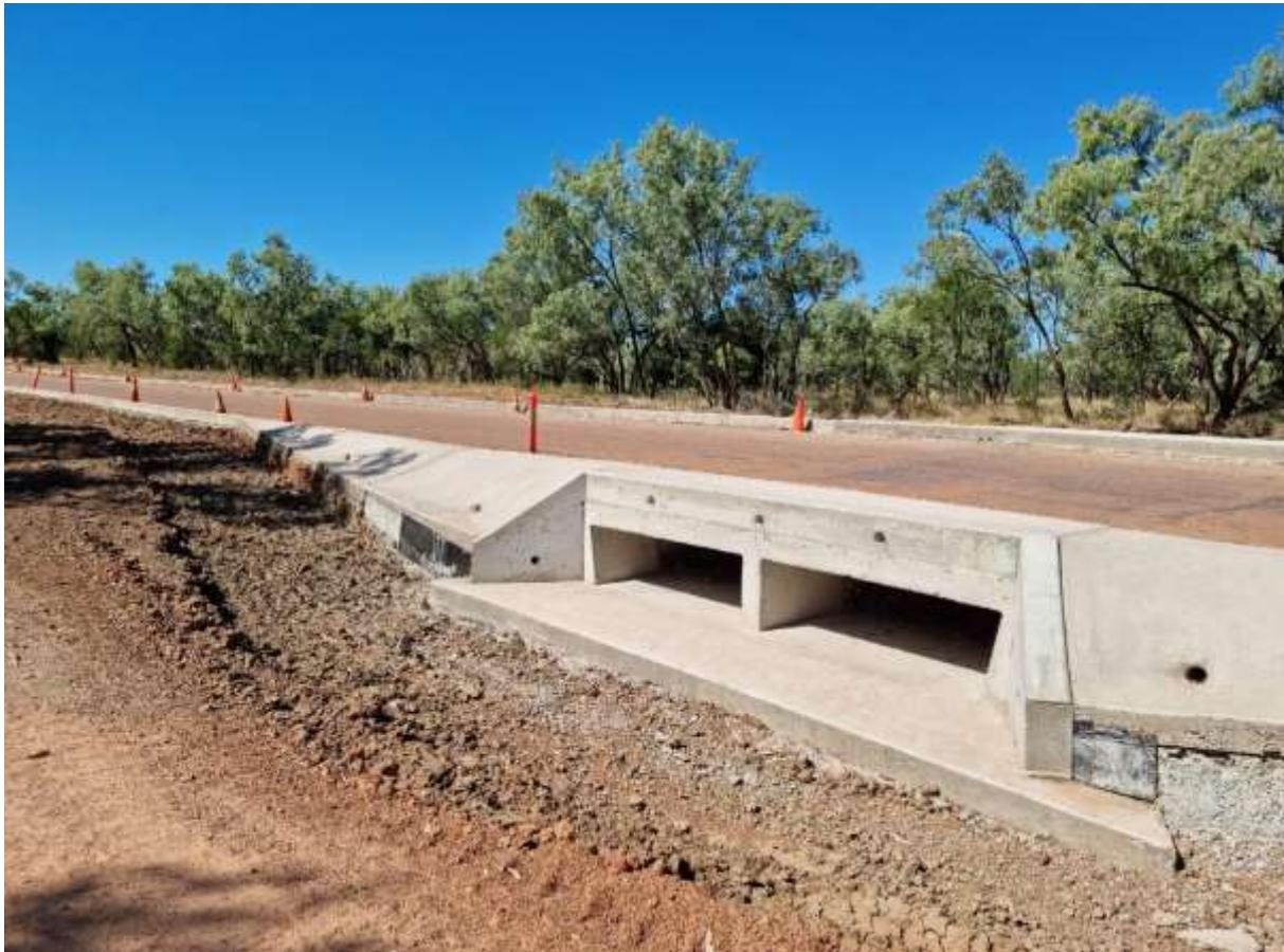
**Photo:** 89A concrete protection works southern end of the Flinders River section.
