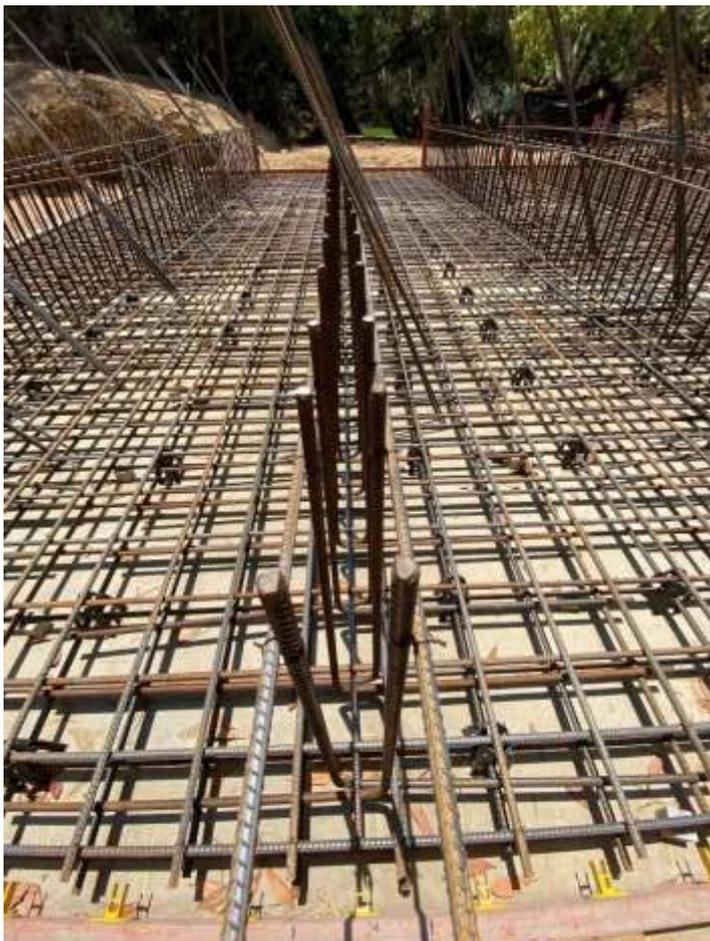
**Photo:** ATSIDIS - Magnificent Creek Overflow (Topsy Ck) – Setting up reinforcement
