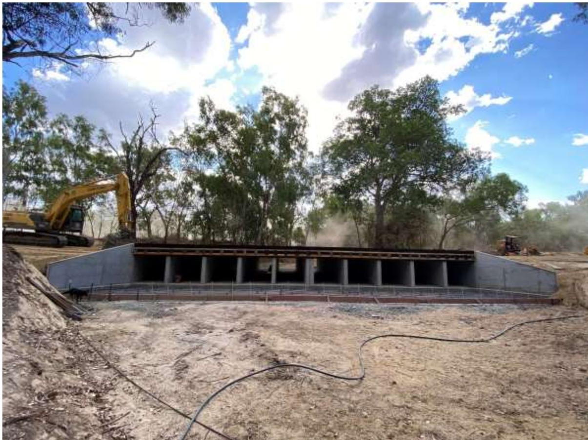
**Photo:** ATSTITIDS - Magnificent Creek Overflow (Topsy Ck) causeway under construction
