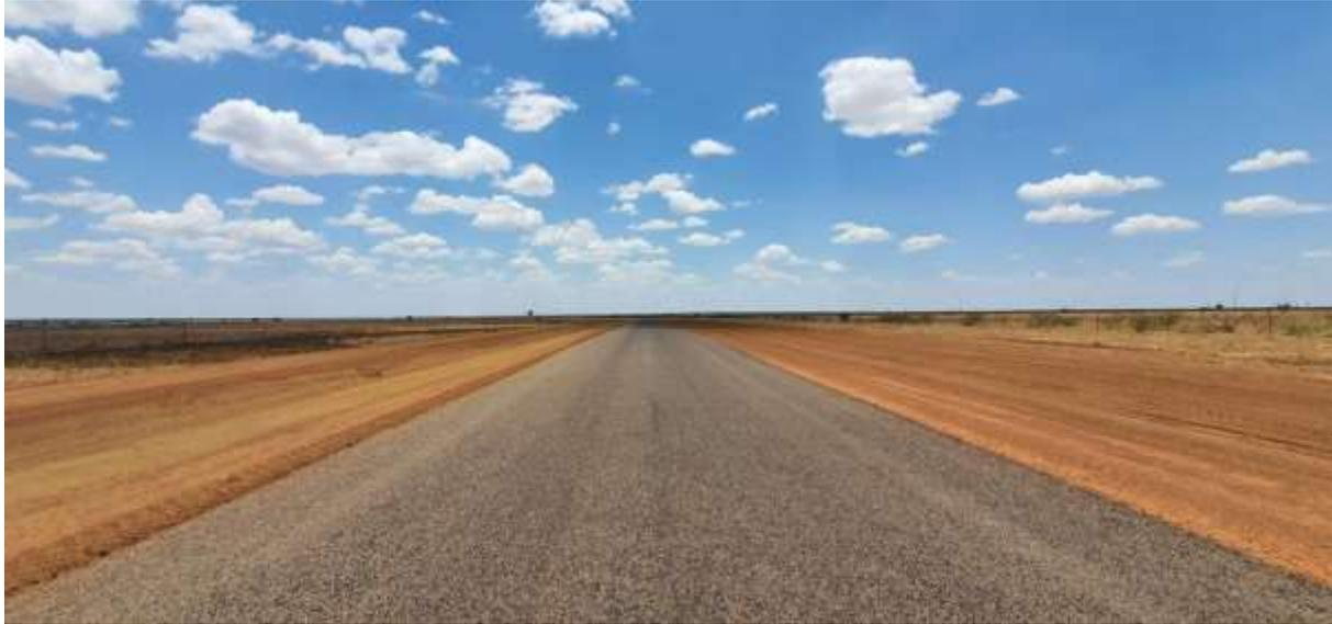
**Photo:** Completed bitumen seal of Betterment Project approximately 5 to 10km west of Inverleigh on the Burketown Road
