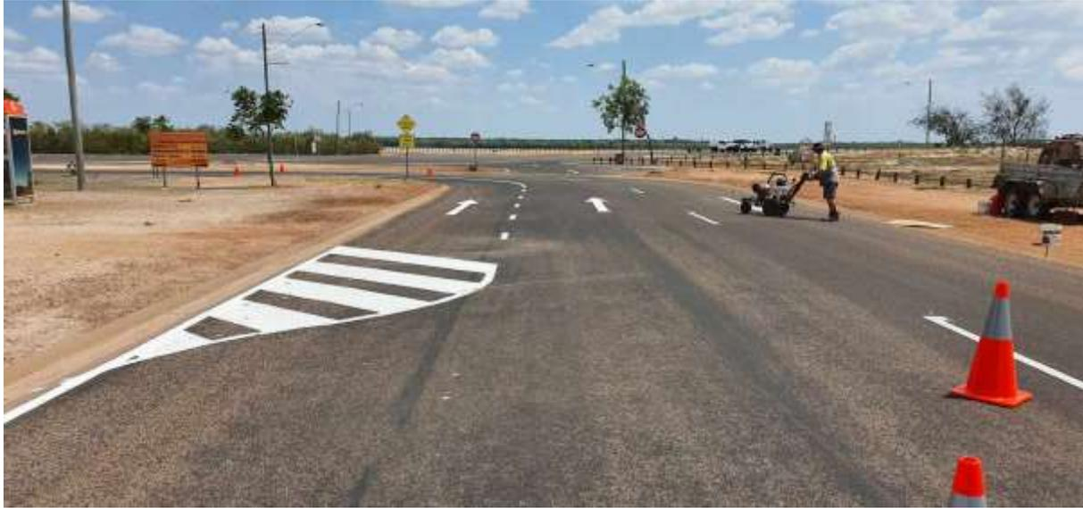
**Photo:** Setting out Linemarking at the Point
