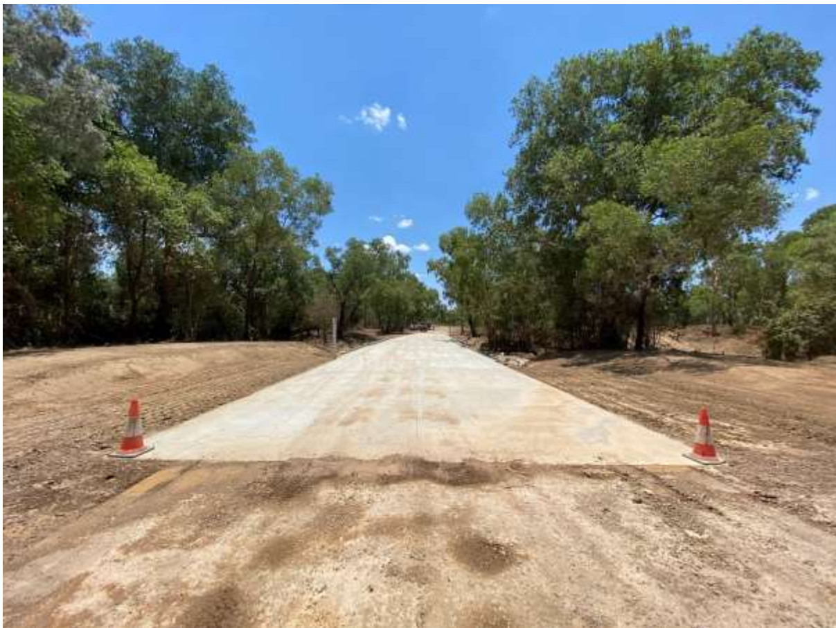
Photo: ATSI-TIDS - Magnificent Creek Overflow (Topsy Ck) – Finished slab approach
