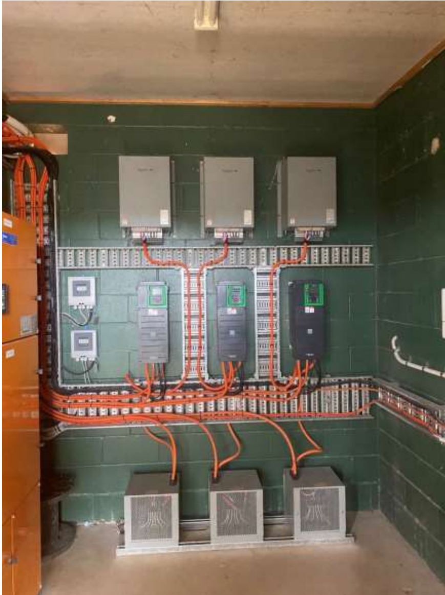
Photo: Glenore weir harmonic filter and flow meter
