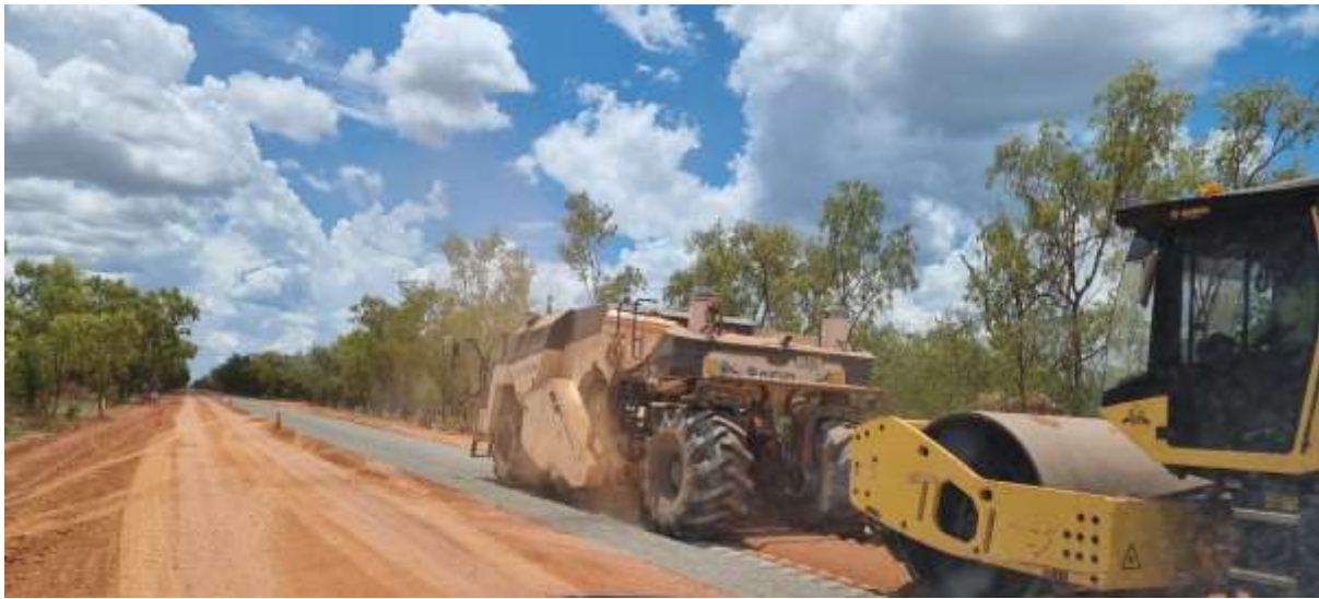
Photo: Pave and Seal AG Stimulus Package 4 on 89B Cement Stabilisation Works
