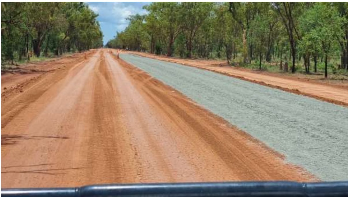
Photo: Pave and Seal AG Stimulus Package 4 on 89B Cement Stabilisation Works
