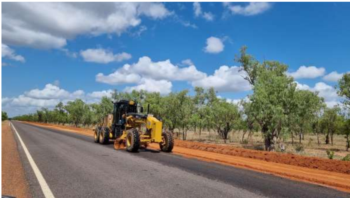
Photo: 2021 DRFA repairing flood erosion at shoulder on 89B
