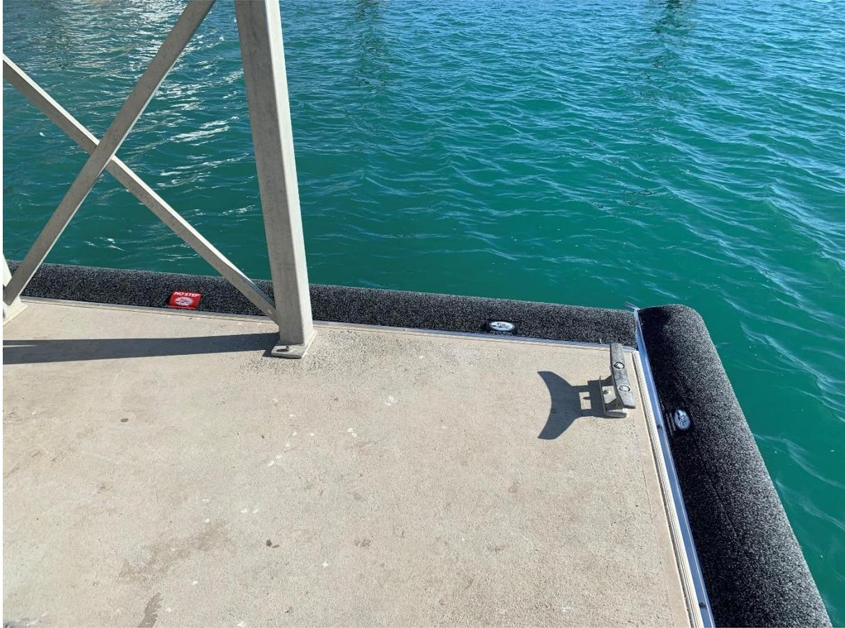
**Photo:** New Fenders at the Karumba Pontoon
