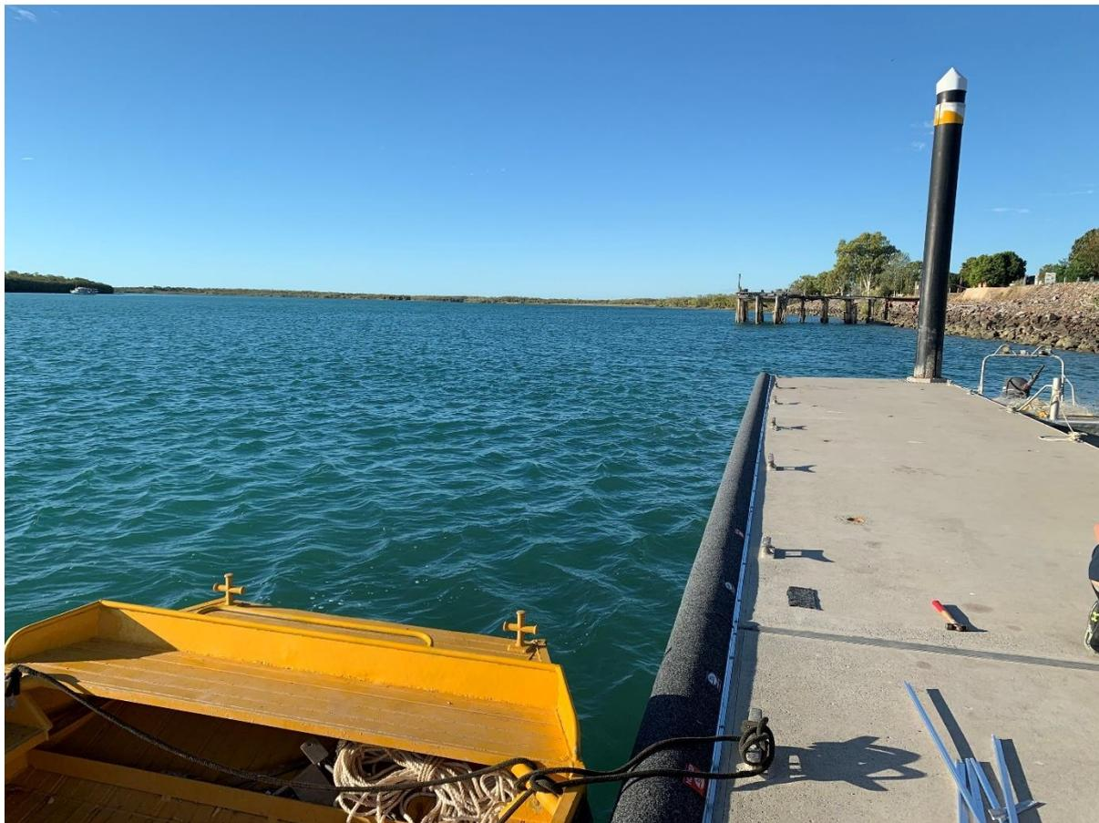
**Photo:** New Fenders at the Karumba Pontoon
