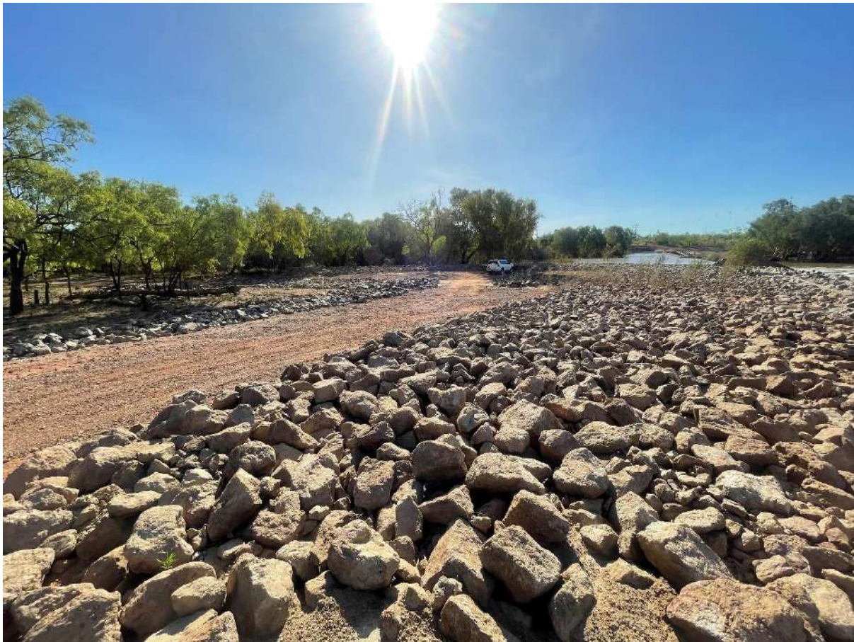
Photo: The rock placement to protect scouring has worked and survived the recent floods.
