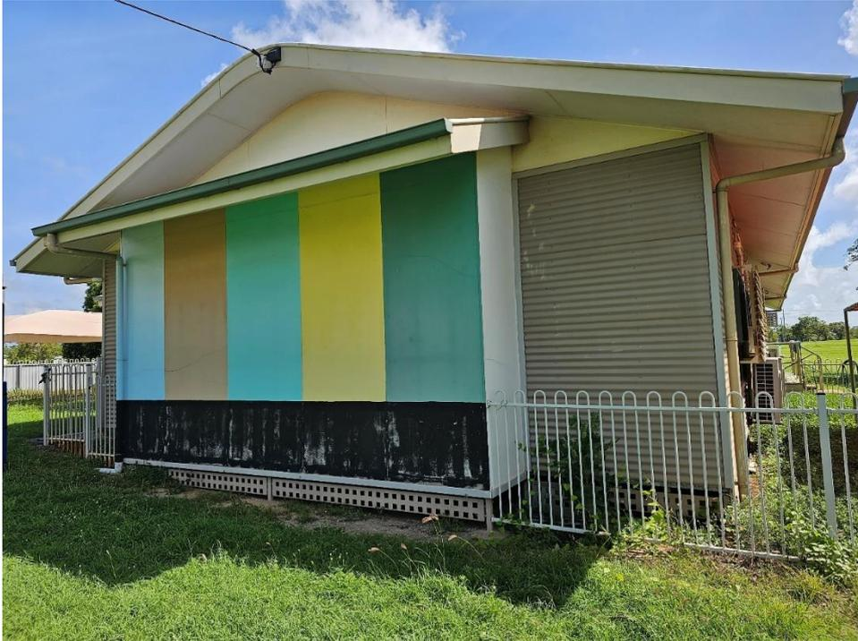
**Photo:** Northern Wall using Fibre Cement Sheets.
