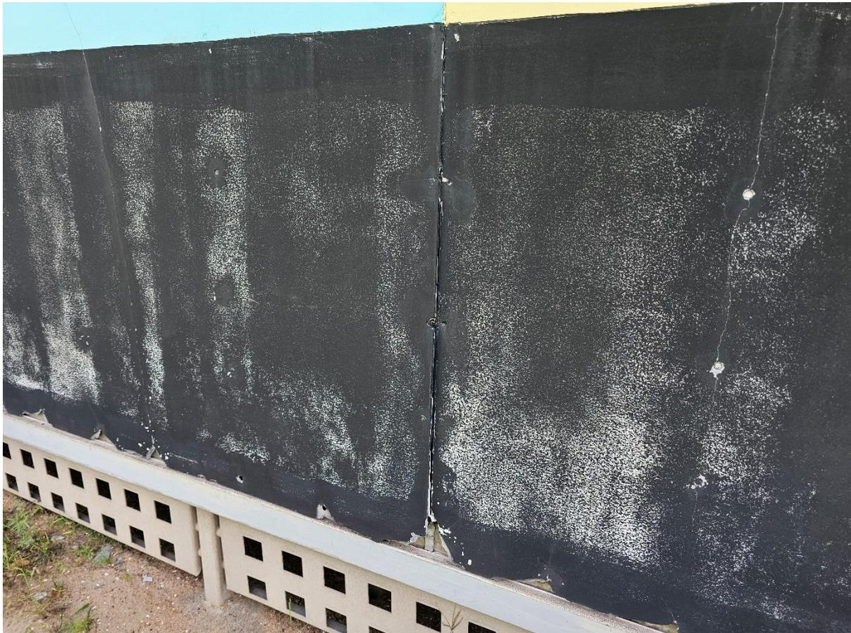
**Photo:** No sealant at the joint causing moisture ingress and minor lifting at the edge.
