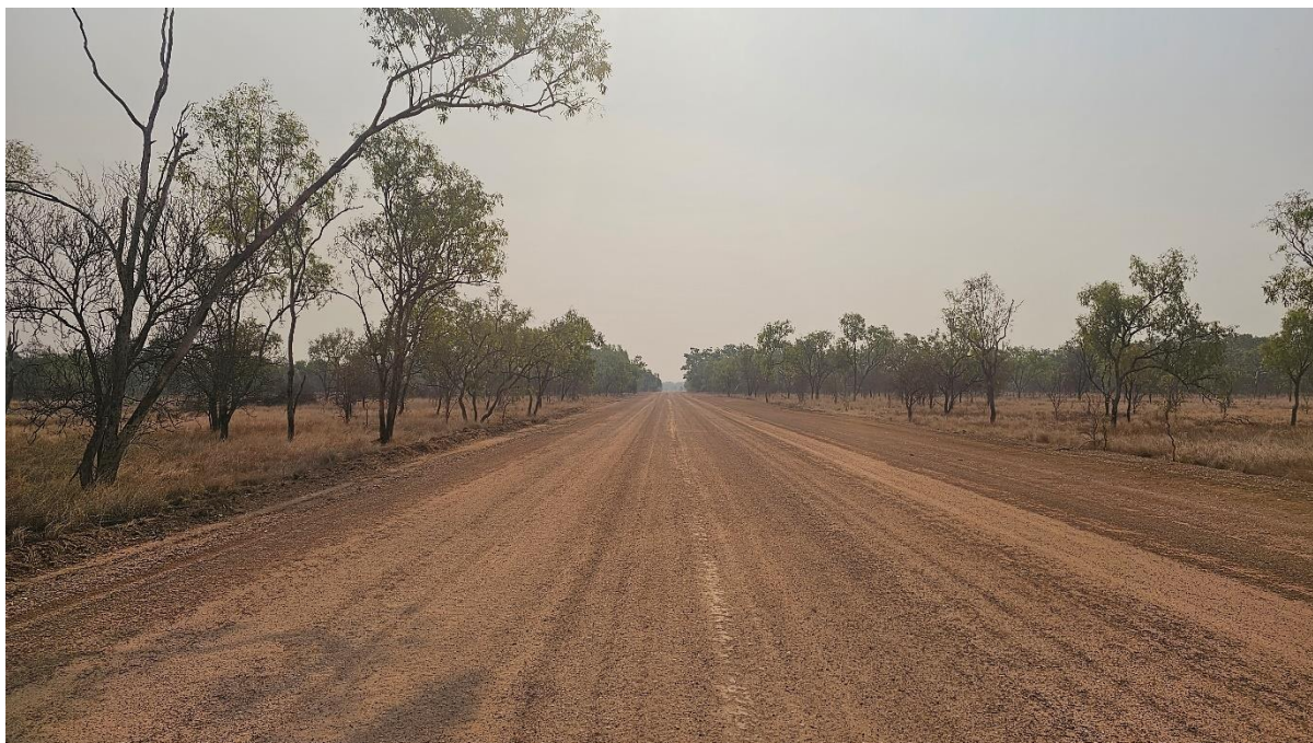
Photo: TMR Betterment Works – Stabilised Works ready for sealing
