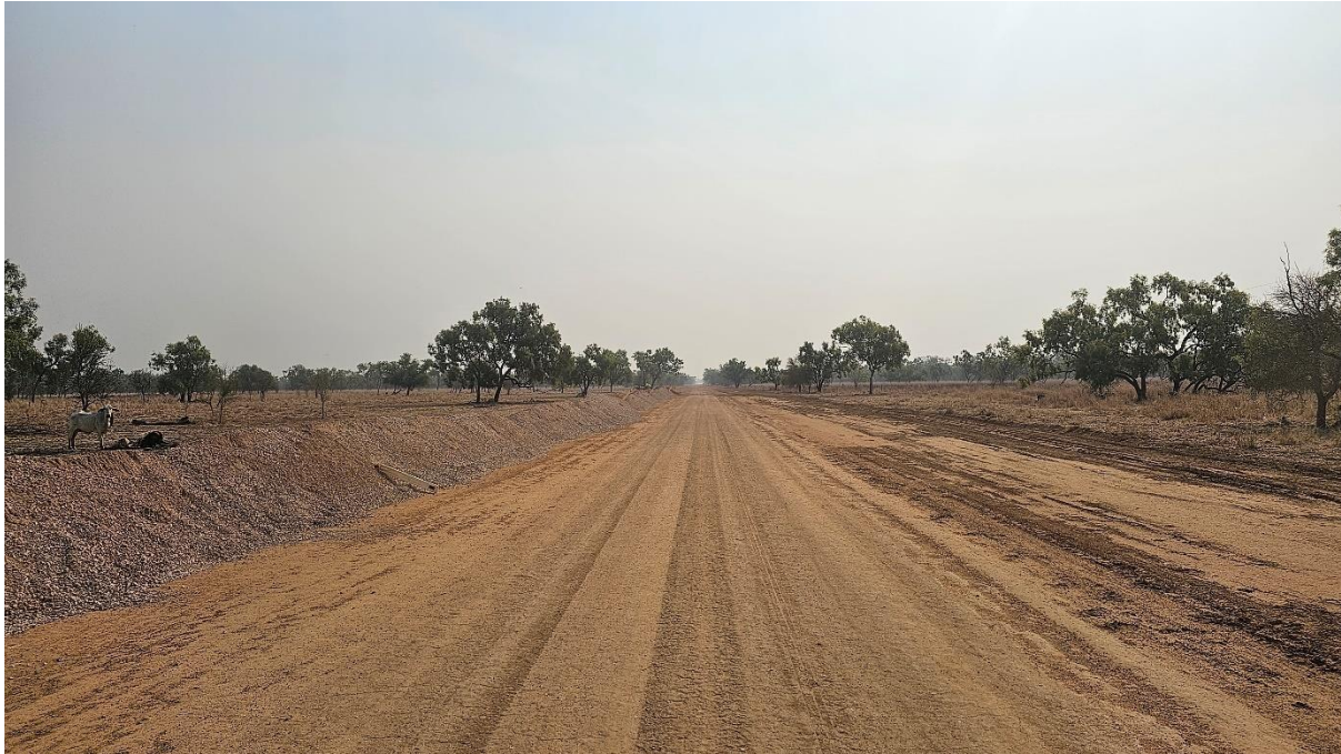
Photo: TMR Betterment Works – Subgrade works
