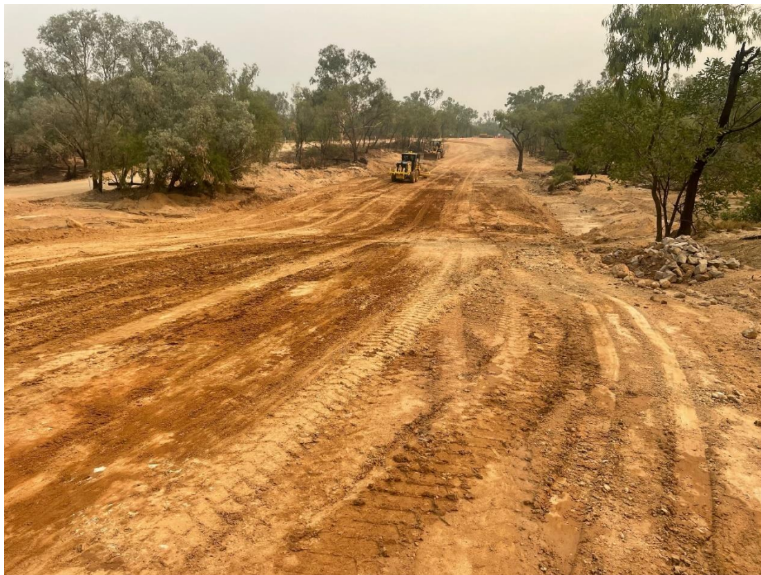
Photo: Clark Creek – Placing gravel over slab to open road
