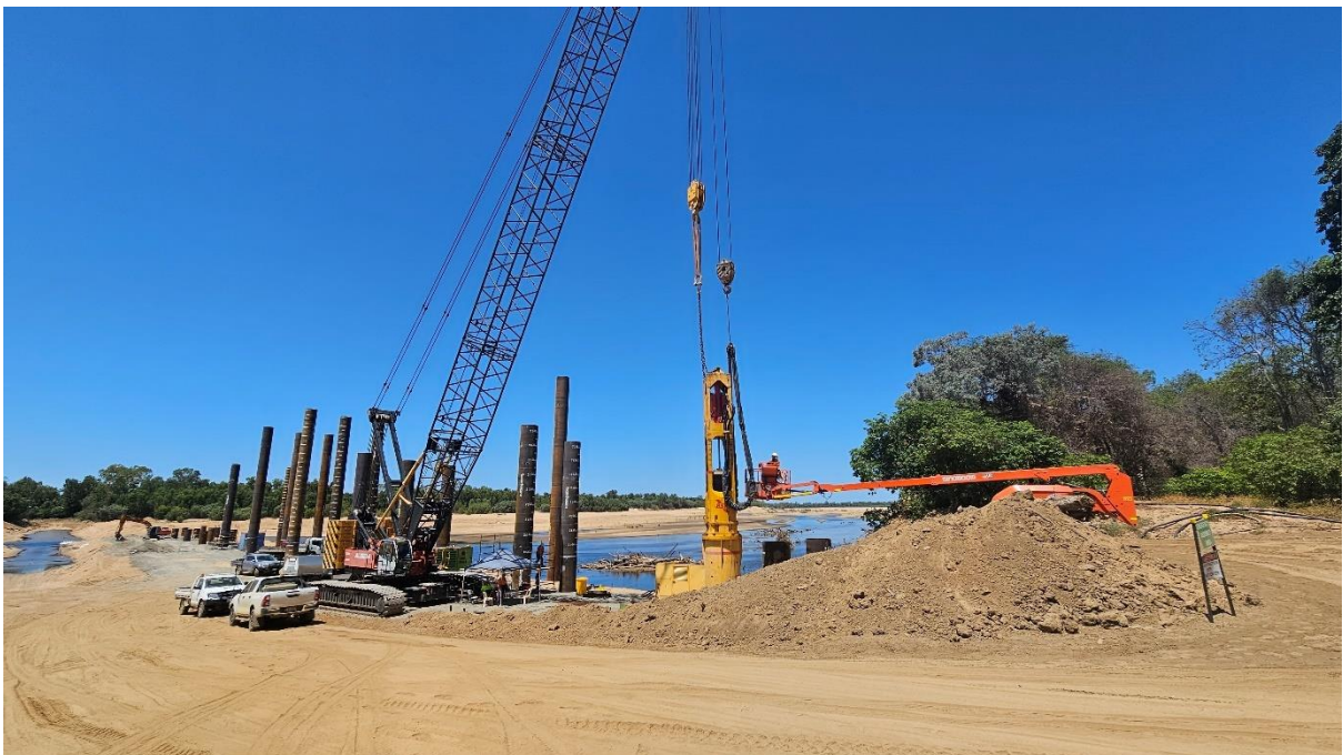
Photo: Mitchell River Bridge – Installation of pile steel liner
