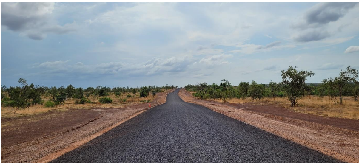
Photo: Burketown Road – 14mm first coat bitumen seal (Inverleigh West)
