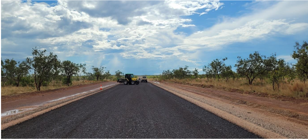
Photo: 10mm second coat bitumen seal – Burketown Road
