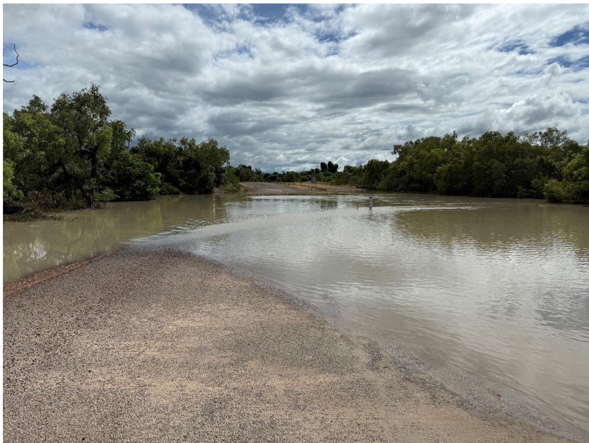
Photo: Flooding at Armstrong Creek – 500mm deep. Before the upgrade it would be around 1.7m deep.
