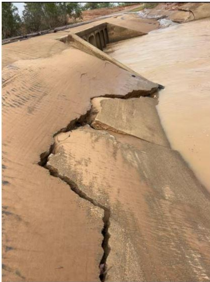
Photo: Damage at M Creek – Was submerged by 2m.
